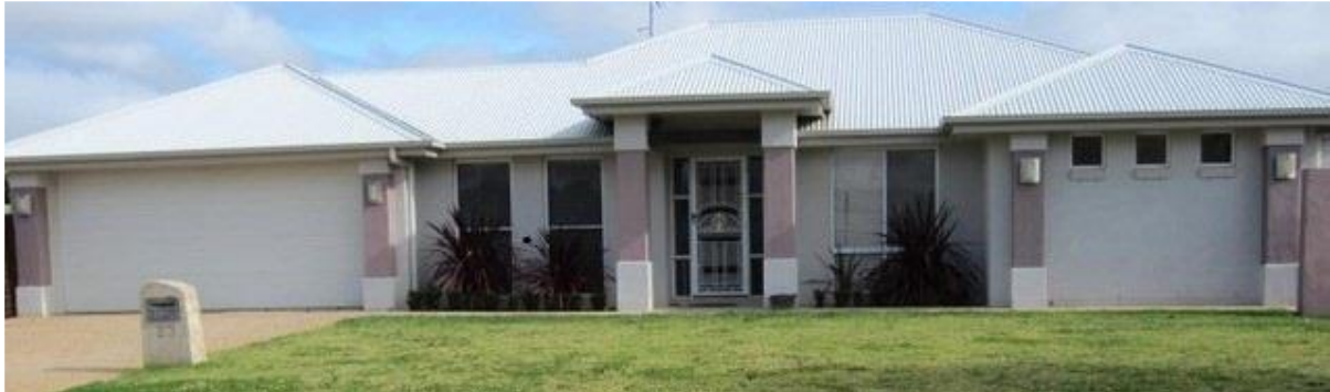
Priest's residence in Highfields.
