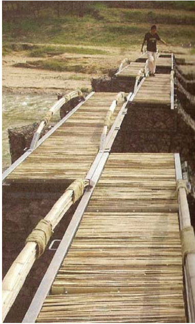
The 'Bridge Too Far' project on the Po River, Maosi, Gansu Province, China is a good example of a simple structure for crossing a flood prone river. (Sinclair & Stohr 2006, p.274)
