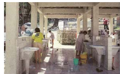
The 'Favela Bairro' program of the 1990s saw a focus on architecture that provided community infrastructure rather than housing. Sports fields (left), community laundries (above), public space and street improvements. This focus, and a participatory process has led to greater success. (Images: Architecture For Humanity , p220)
