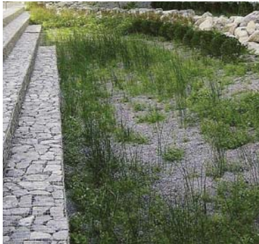
Above: A simple rain garden to slow and treat water also becomes an important element in a park.
