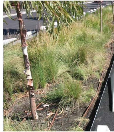
A vegetated bioswale in Victoria Park, Sydney. This swale captures stormwater, slows it down and the plants remove pollutants. These swales become important green elements in the streets.
