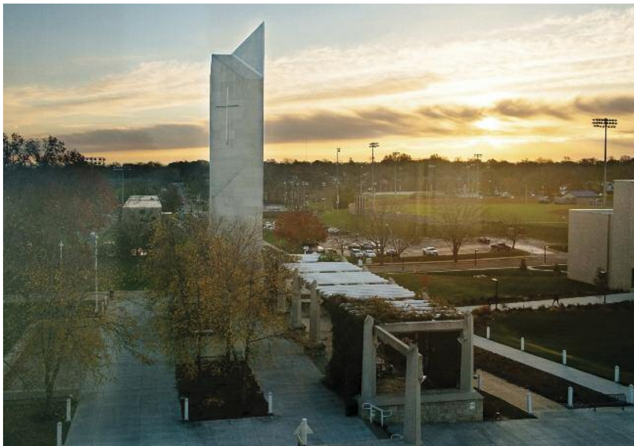
The campus bell tower. Photos courtesy of Rockhurst University.
