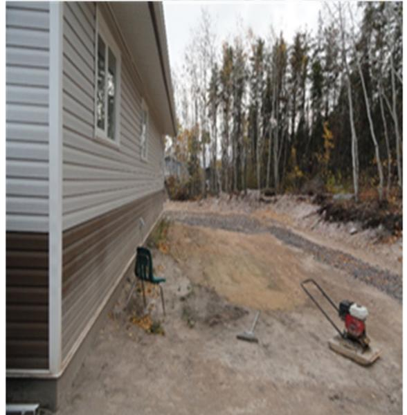
Before and after pictures showing the addition of a French drain. Before the addition of a drainage ditch, the house was chronically flooding in the spring or during heavy rains. The basement is now dry and the occupants are developing the basement.
