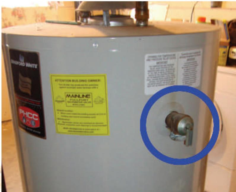
*Note the build-up on valve and lack of valve stem.*
