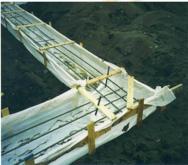
Lumber-form strip footings are installed similarly. First, the strip footing location is identified, stakes are driven into the ground and 2x4 s are attached to the stakes at the top of the strip footing. Next, a strong flexible interwoven fabric is laid out and secured between the formwork. The concrete is placed, leveled and allowed to set. Since the formwork is protected from the concrete, it can be re-used, often without having to be cleaned.
