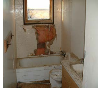
Figure 3 Repairs to bathroom
