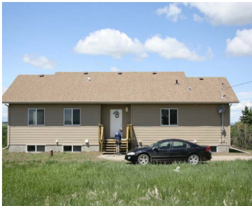
Figure 9 A home in a community that emphasizes building homes to code and other standards.
