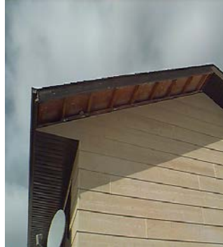
Figure 2 Repairs to Soffit
