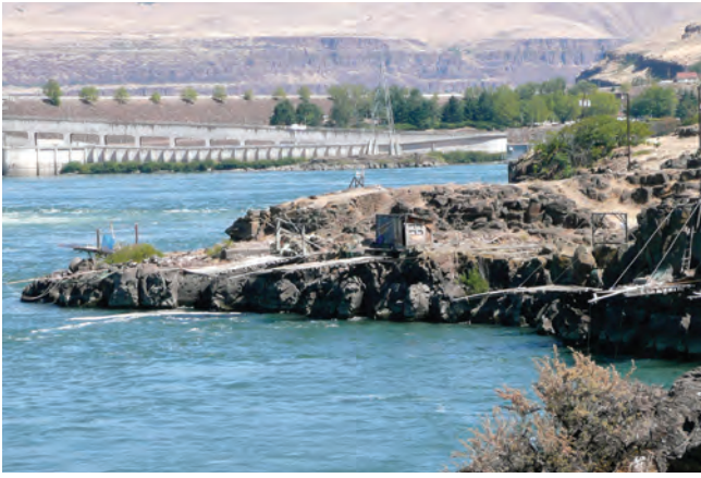
Fishing platform across from The Dalles Dam, Source: CRITFC
