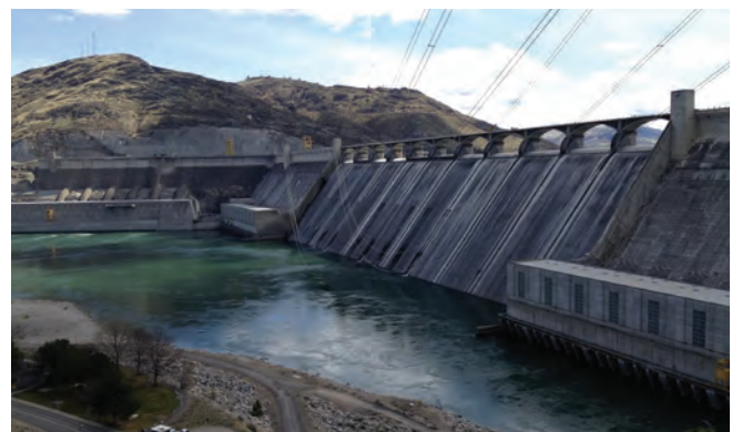
Grand Coulee Dam , Source: CRITFC
