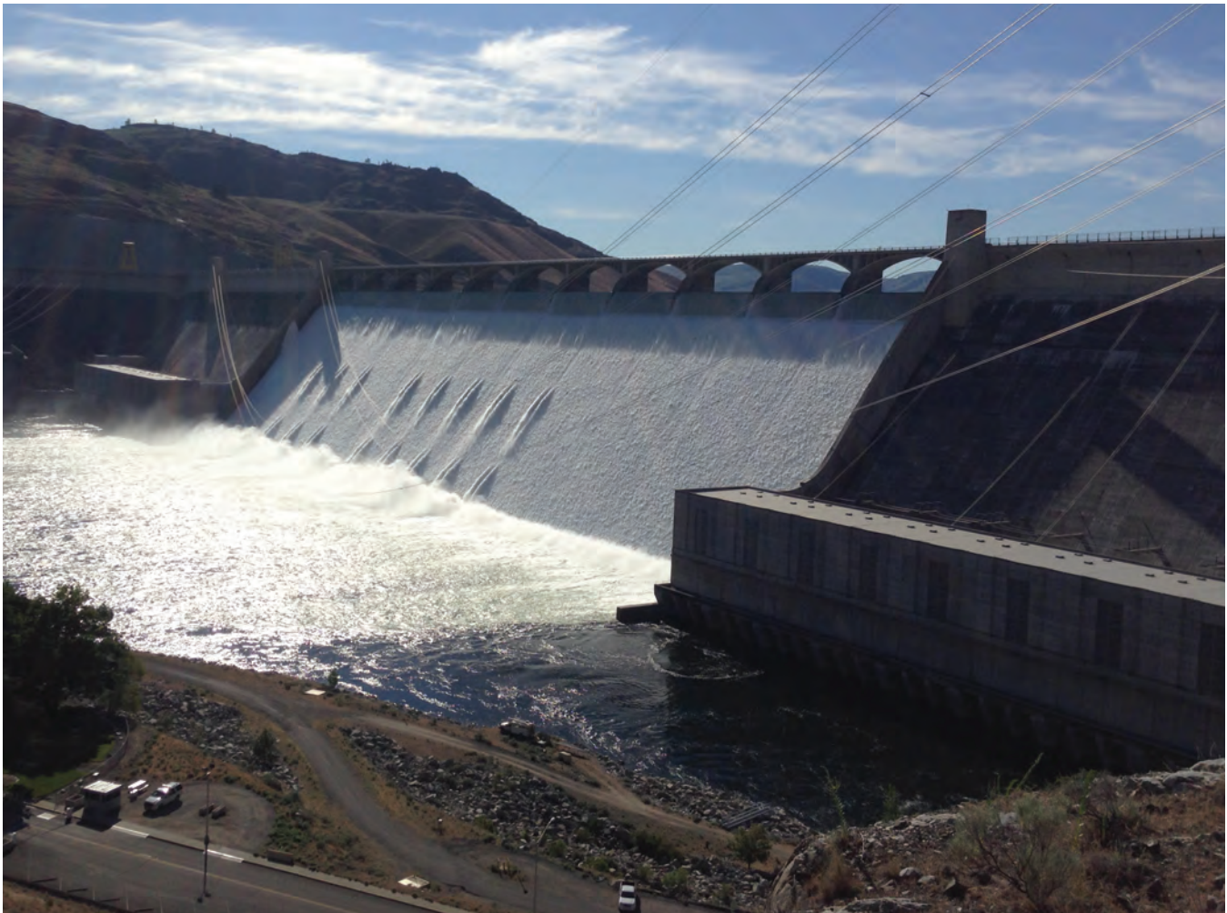
Grand Coulee Dam, Source: Keith Kutchins
