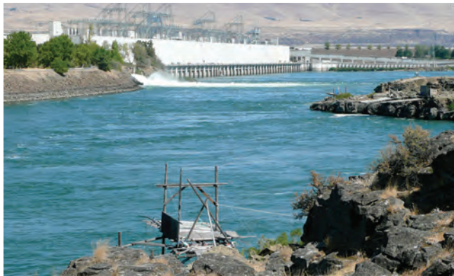
Fishing platform across from The Dalles Dam, Source: CRITFC
