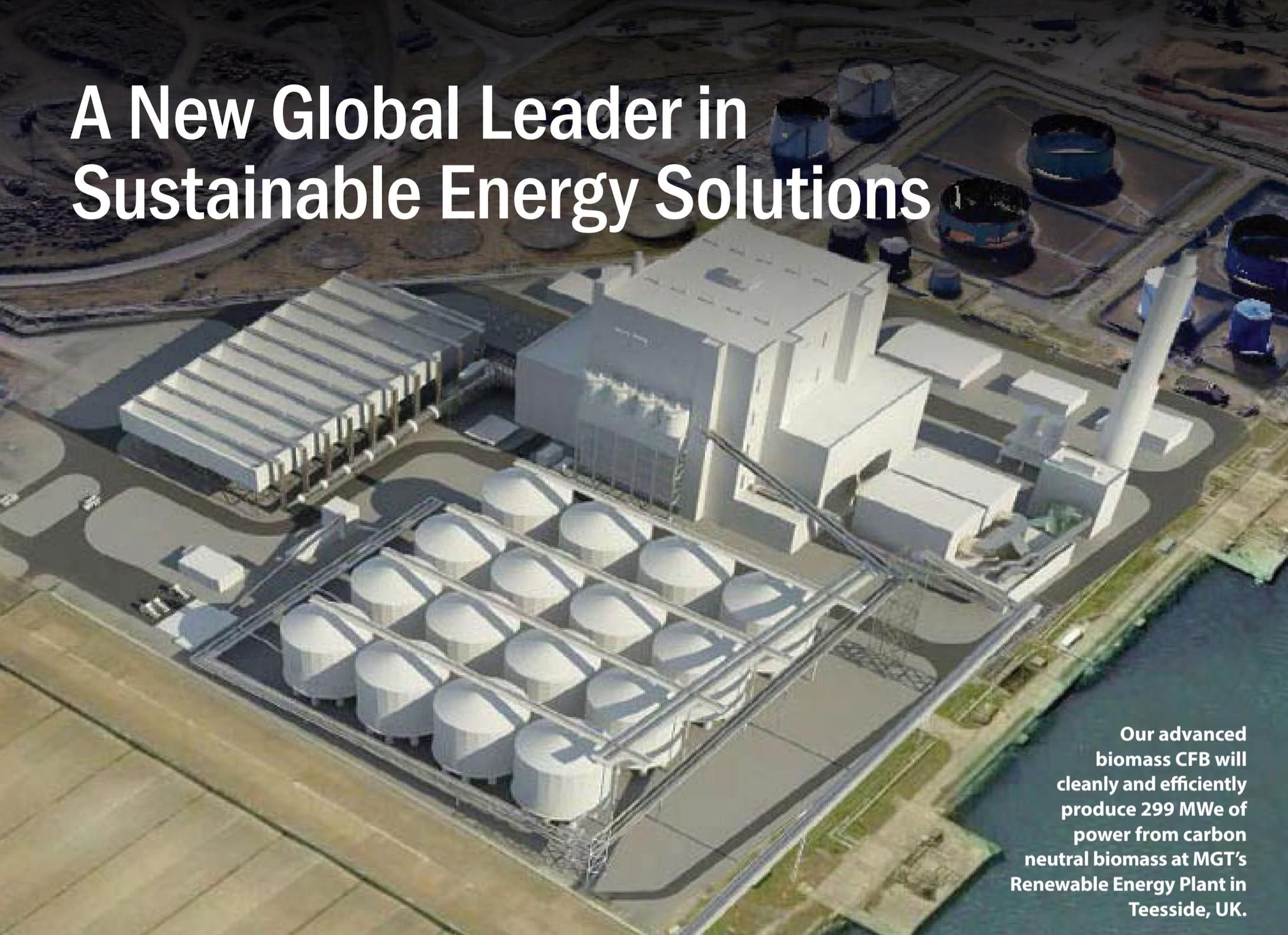
Our advanced biomass CFB will cleanly and efficiently produce 299 MWe of power from carbon neutral biomass at MGT's Renewable Energy Plant in Teesside, UK.
