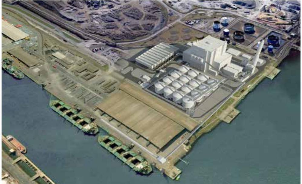
When commissioned in January 2020, the 299-MWe Tees Renewable Energy Plant will become the largest 100 percent biomass-fired power plant in the world. The Teesside plant is built around a Sumitomo SHI FW CFB boiler and a single steam turbine, along with a fuel storage area and conveyor system, a woodchip drier, and air-cooled condenser.
