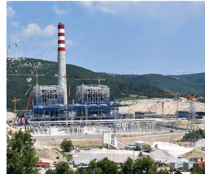
The 510 MWe Soma Power Plant is the largest CFB project ever awarded in Turkey and features two of Sumitomo SHI FW's CFBs.
