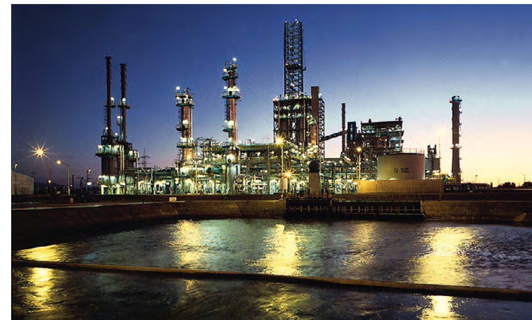
Sumitomo SHI FW built the 74 MWe cogeneration facility at the Petropower Plant in Talcanuano, Chile, which has been successfully operating since 1998.
