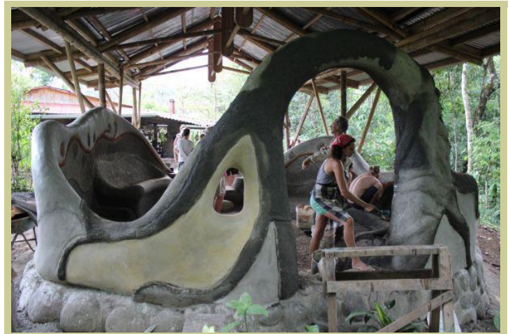
Lime Plastering the Lounge
