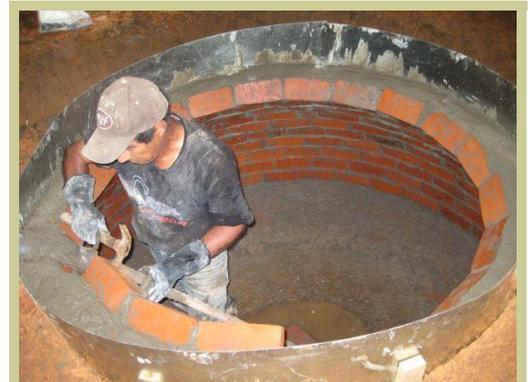
*Jose Luis Zuniga doing the brick work for the Ranch's methane biodigester*
