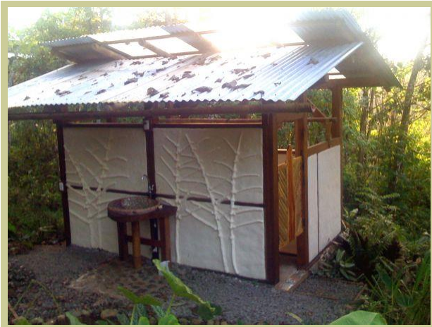
The new shower house at Rancho Mastatal photo by Ian Woofenden
