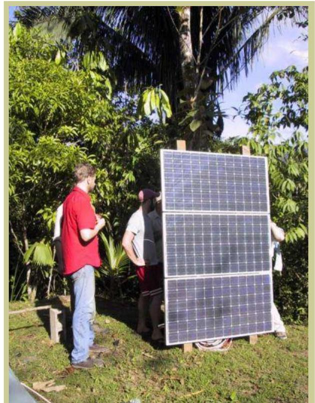
*Photos from an SEI class in January 2006. Testing the solar panels before they go on the roof
