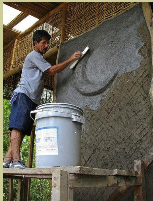
Gilberth applies a lime plaster to an exterior wall
