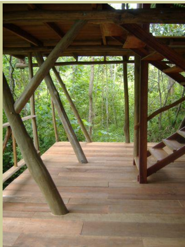
Hankey House first floor staircase
