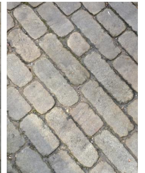
Figure 3.16: Tumbled Yorkstone setts to parking bays on Park Lane Street
