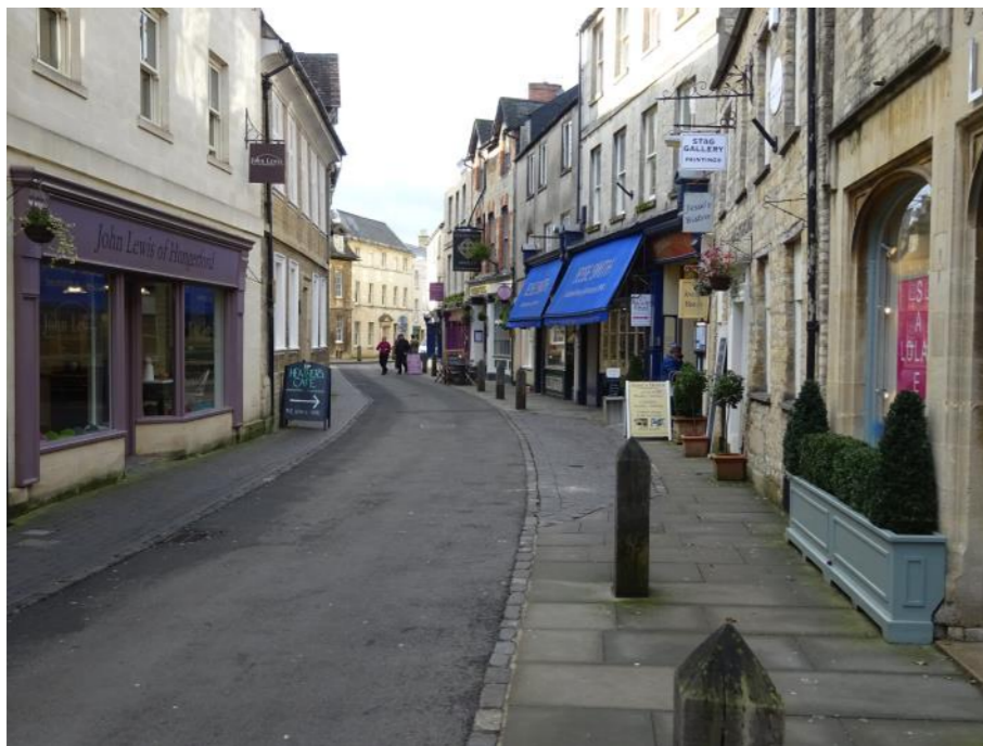
Figure 3.13: Yorkstone flags, granite setts and blue brick paving on Black Jack Street
