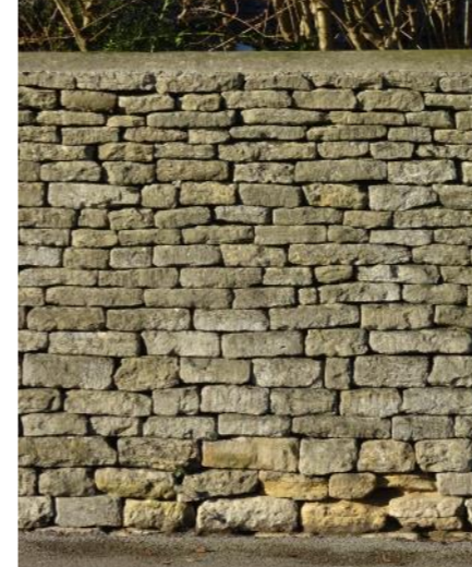
Figure 3.53: Cotswold 'dry' stone wall with rounded concrete capping on Spitalgate Lane
