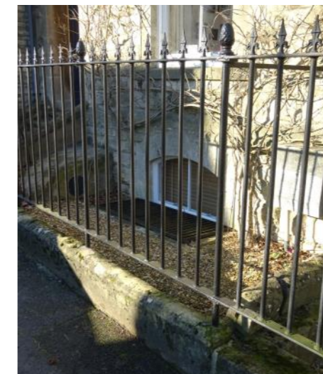
Figure 3.56: Metal Railings on top of a low stone wall on The Avenue
