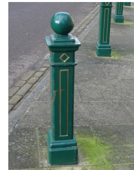
Figure 3.24: Square section cast iron bollards on Park Street
