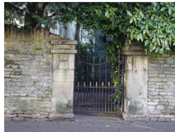
Figure 3.54: Pointed Cotswold stone wall with 'cock-and-hen' coping on Watermoor Road
