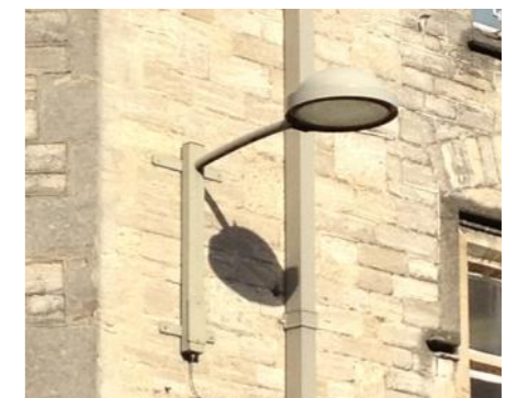
Figure 3.44: Wall mounted version of the contemporary half spherical lantern, painted cream to match the local stone on Castle Street
