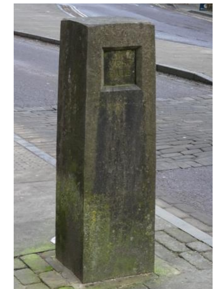
Figure 3.25: Square section stone bollards act as a gateway feature at the western end of Castle Street
