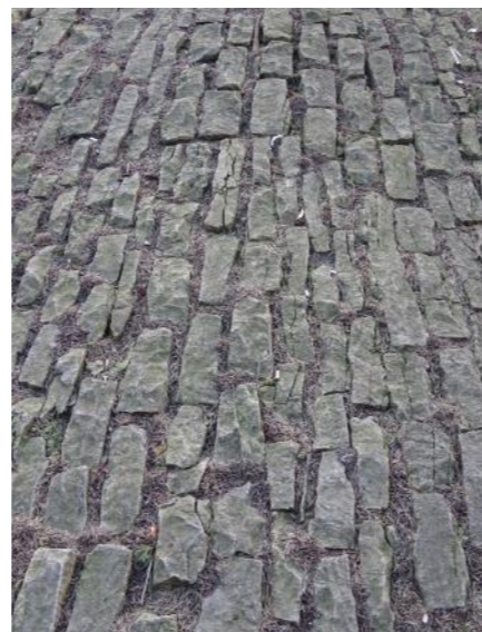
Figure 3.1: Limestone setts in Gosditch Street
