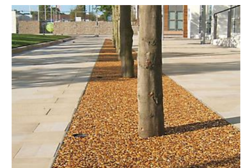
Figure 3.50: Porous resin bound gravel tree pit surfacing. Image shows 'Addastone TP' from Addagrip
