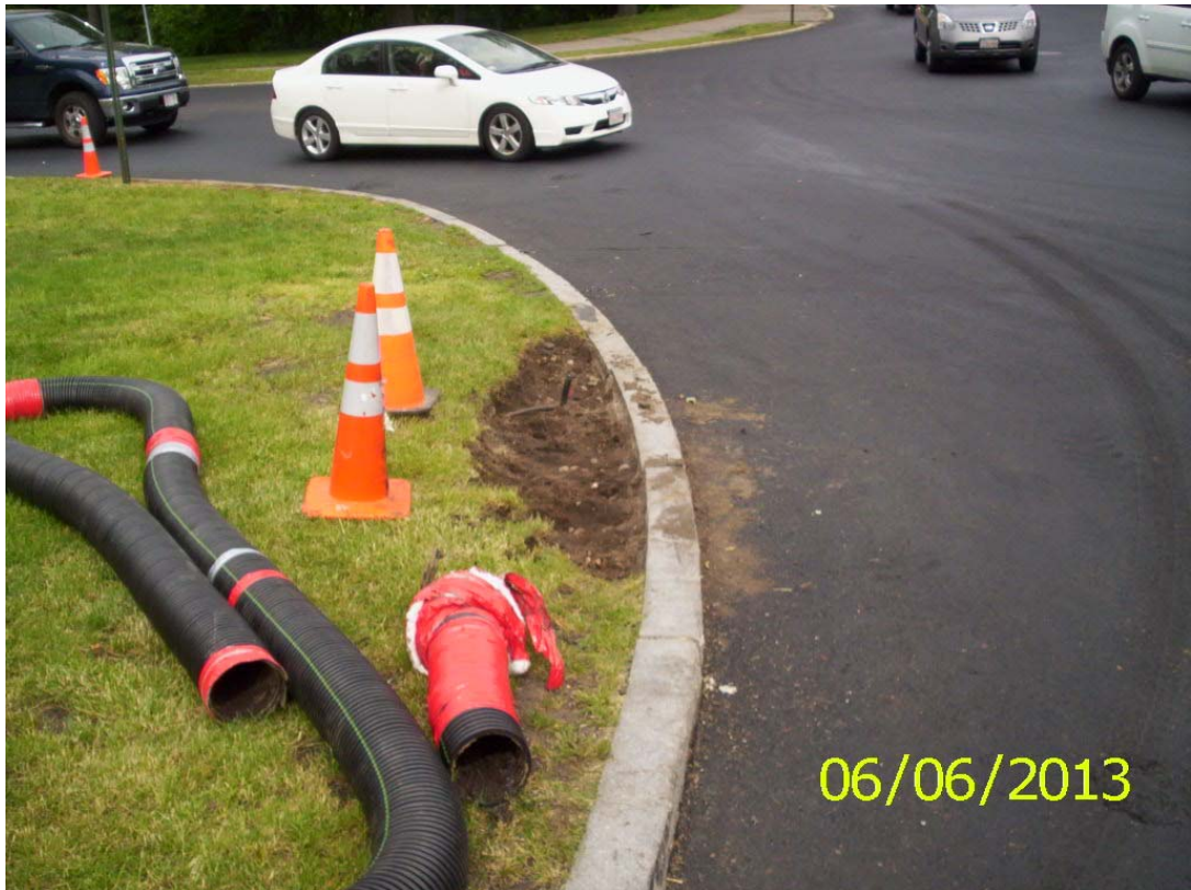
Photograph 18: View of completed excavation adjacent to rotary. Photograph taken on June 6, 2013.
