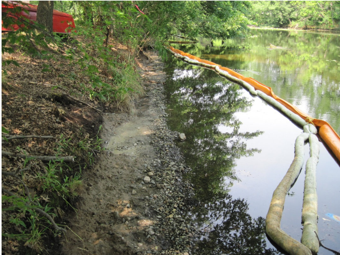
Photograph 20: View of station 1450-1550 (Boom 2 Collection Area, 1485') during removal of impacted sediments/moss and water washing. Photograph taken on June 25, 2013.
