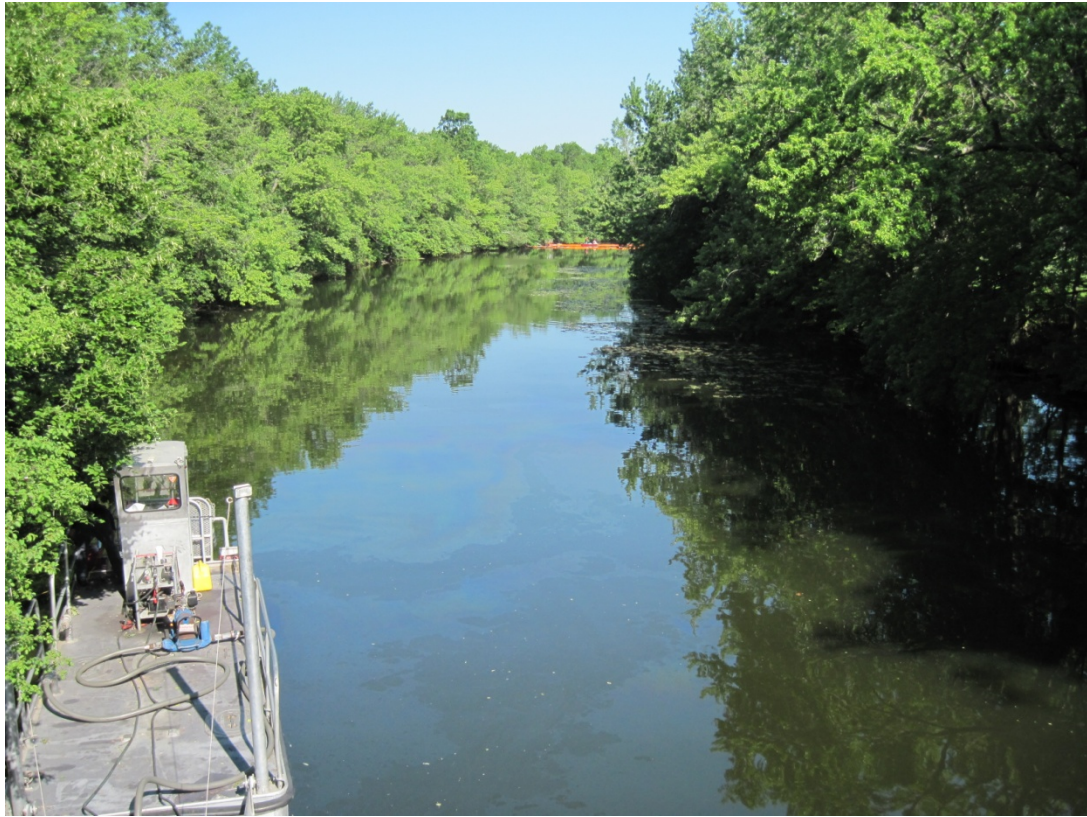
Photograph 9: View of Mystic River from River Street bridge facing upstream. Photograph taken on June 2, 2013.
