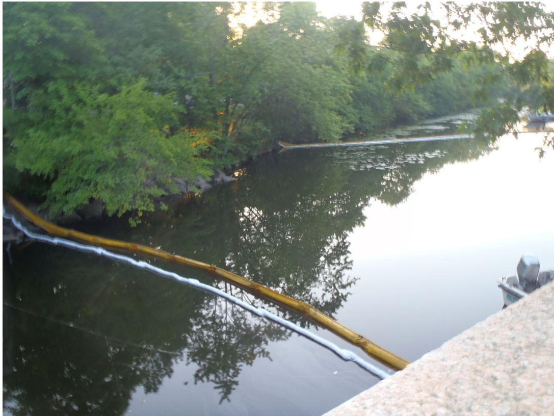
Photograph 6: View of containment boom deployed in Mystic River below River Street bridge. Photograph taken on June 1, 2013.
