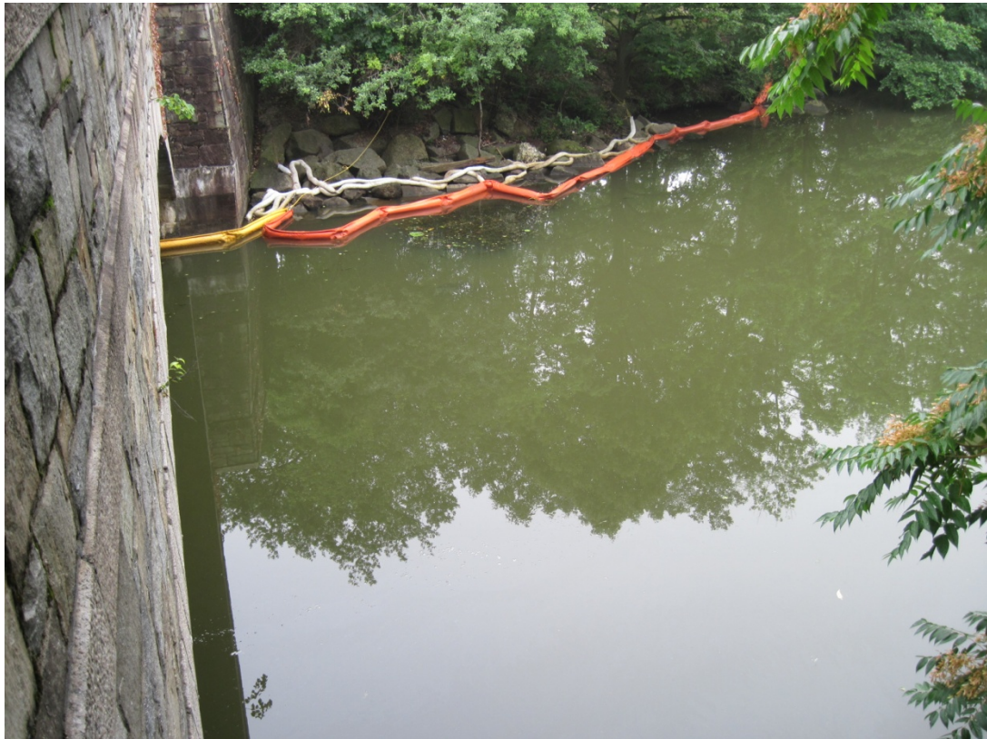
Photograph 30: View of absorbent and containment boom at station 2657 to 2682 (rip rap to River Street bridge). Photograph taken on July 10, 2013.
