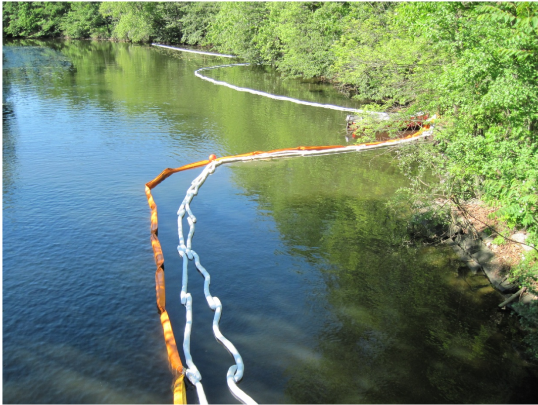
Photograph 15: View of absorbent and containment boom at Medford Street bridge during water washing and shoreline cleanup. Photograph taken on June 5, 2013.
