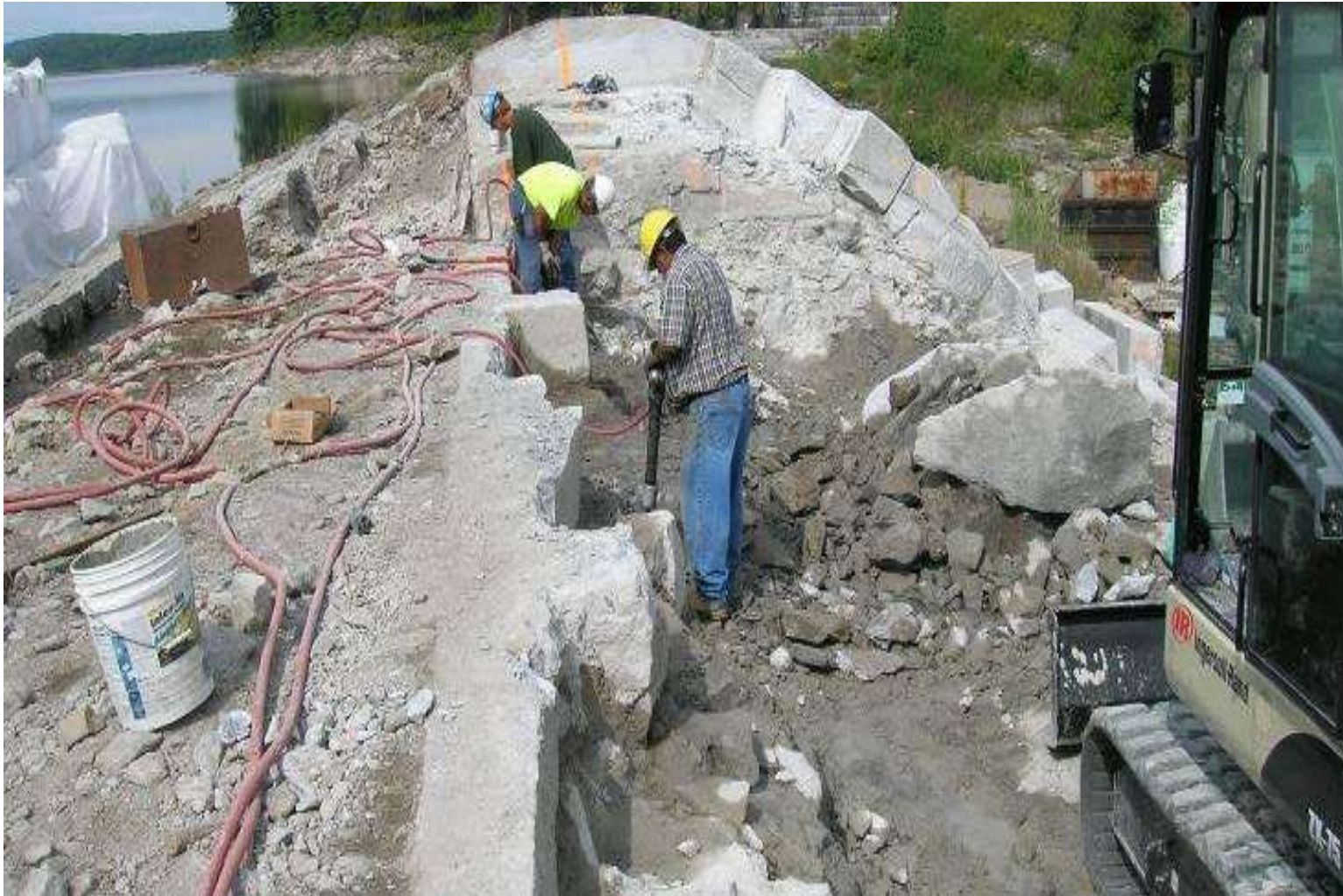
Wachusett Spillway capacity increased by lowering it 2 feet
