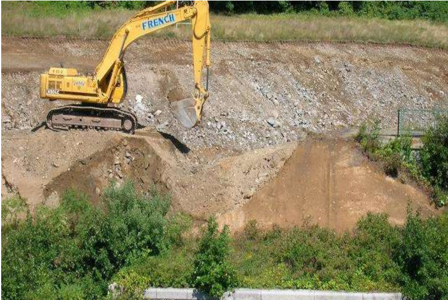
New Wachusett Auxiliary Spillway constructed to pass flood discharge
