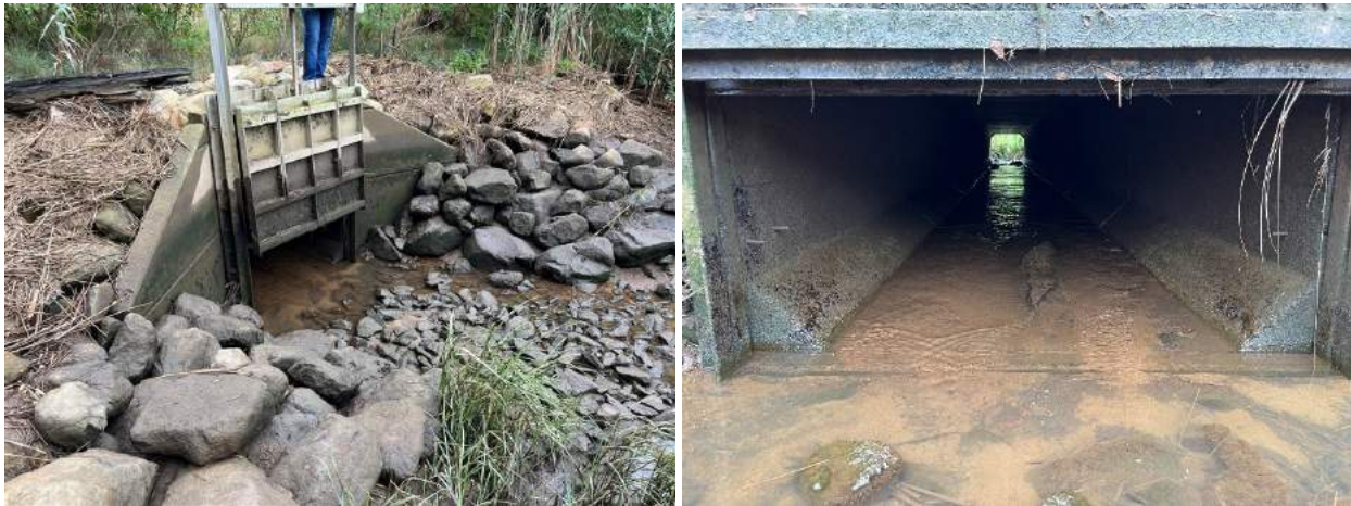
Figure 56. Example of weir boards on the face of a large culvert used for water control in Orleans, MA.
