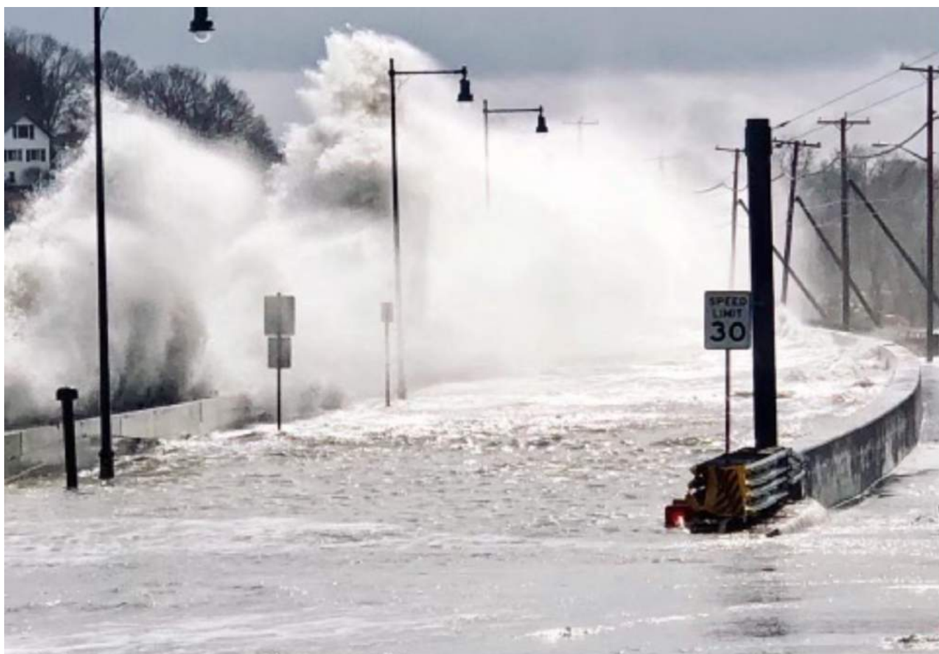
Figure 5. Wave overtopping and flooding of the Winthrop Parkway during the March 2018 nor'easter. Source: WBUR, photo courtesy of Sandra Castellarin.
