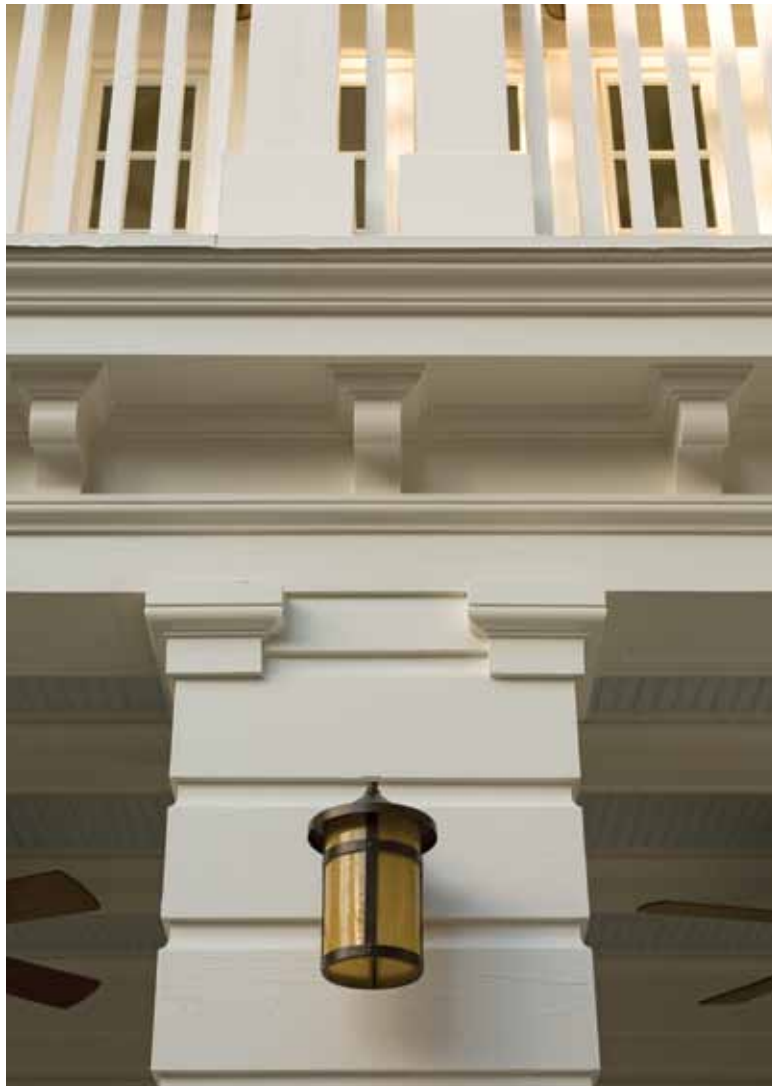
Drawing on a Carpenter Gothic tradition employed in many southern locales, the belt course is animated with brackets in the form of bird's beaks.
