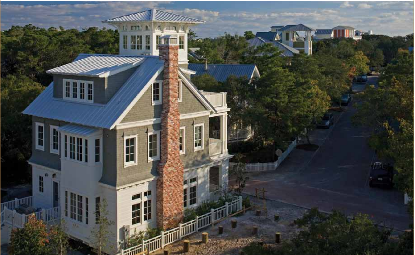
The new 3,000-sq.ft. “57 Malvern” house in Seaside, FL, was designed by Braulio Casas Architects to fit into the urban context of the New Urbanist town while drawing on the owner’s English roots. All photos: Jack Gardner
