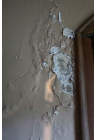
Figure 9.7: Blistering on Chancel Wall; Figure 9.8: Blistering on Vestry Wall. Joseph Newman and Fallin Steffen
