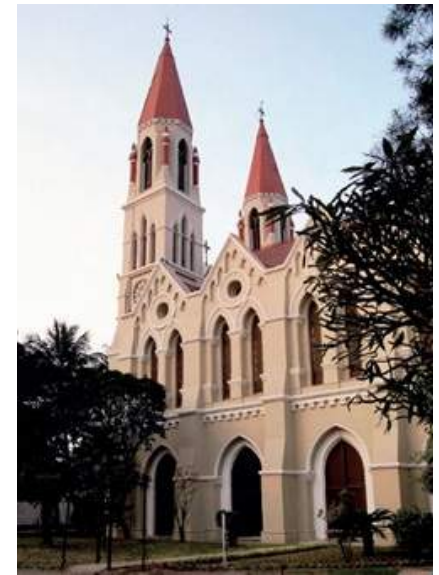
Figure 2.21 Picture of St. James Church in Kolkata, post-restoration work. Photo credit to Manish Chakraborti.
