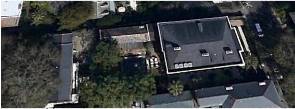
Figure 4.26: Roof of 21 Legare Street 2014 Source: Google Maps, Accessed March 5, 2015.
