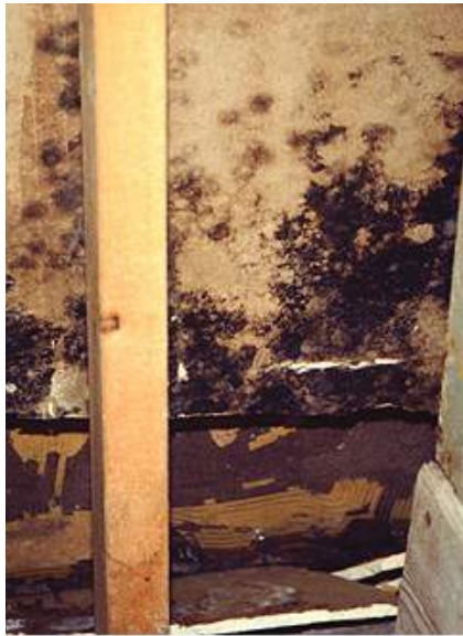
Figure 2.20 Photo of Stachybotrys mold infestation on the backside of gypsum board. Photo credit to Home Improvement Solutions.
