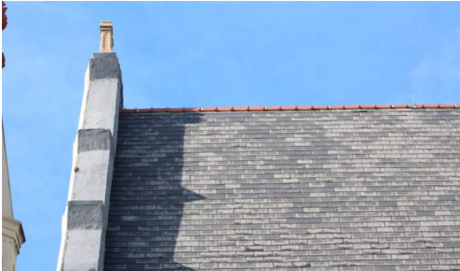
Figure 4.4: Parapet wall at the front of the cathedral. Photo by Cody Ellis, 2015.
