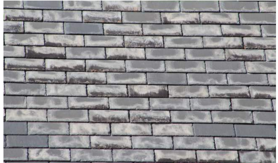
Figure 4.14: Slate shingles on cathedral roof. Photo by Cody Ellis, 2015.
