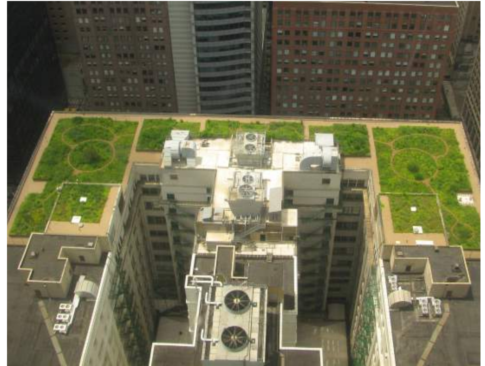
Figure # 6.11: Chicago City Hall has an extensive green roof system. Image courtesy of Tony Tiger and Wikimedia Commons, 2008.
