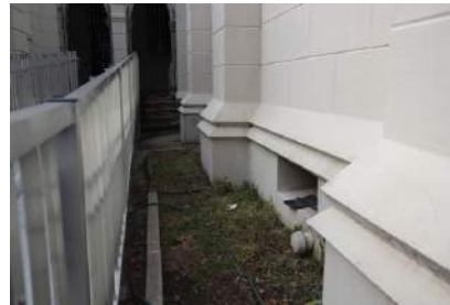
Figure 7.12: "Sacrificial" spot for wheelchair ramp, no landscaping, photo by Amanda Keith, 2015
