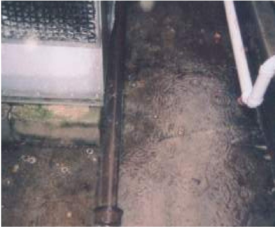
Figure # 6.5: Standing water in the downtown Mechanical Yard. Photo by Dimitri Roby, 2015
