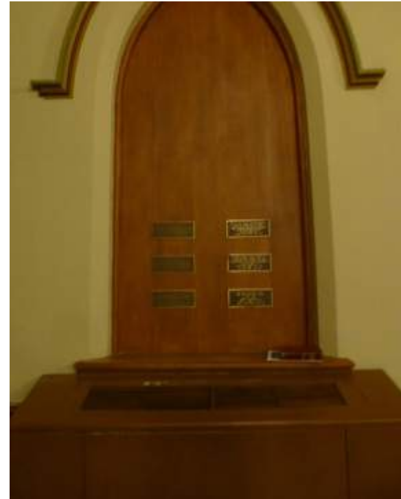
Figure 3.6: Wooden board where stained glass window used to be
