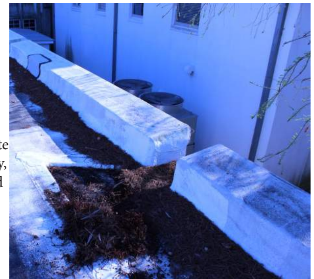
Figure 4.31: Current build up on flat roof overlooking courtyard Photo Christine Carlo, 2015
