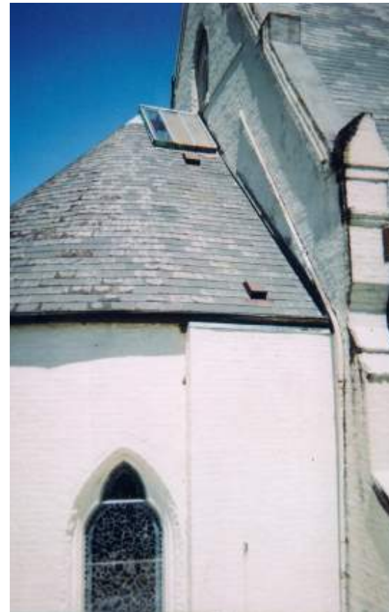
Figure 4.23: Apsé roof. Photo by Cody Ellis, 2015.
