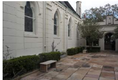
Figure 7.13: The Cloister Garden, view towards St Charles Ave, photo by Amanda Keith 2015
