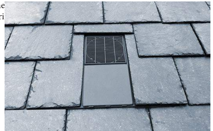
Figure 4.38: Low profile slate roof vent Source: http://www.glidevale.com/2012-07_compact_inline_vent.html
