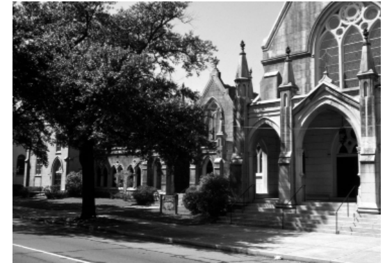
Figure 2.4: View of St. Charles Avenue elevation showing staining on the facade, 1972. Tulane School of Architecture, New Orleans Virtual Archive.
