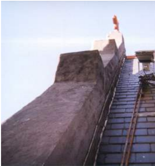
Figure 4.18: Tarred flashing by parapets. Courtesy of Dimitri Roby, 2014.
