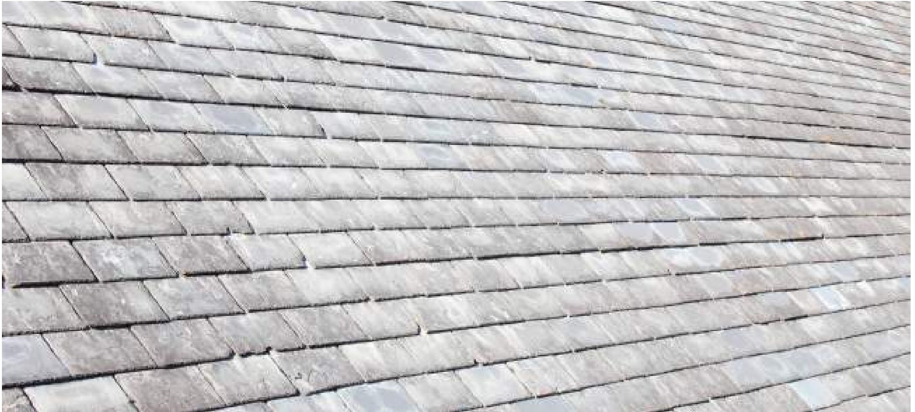
Slate Shingles of Cathedral Roof. Photo by Cody Ellis, 2015.
