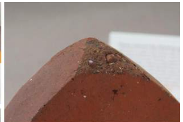
Figure 5.34-5.36 : Ridge tiles on the chapel; mortars and connections noted. Photo by Laura Stokley, 2015
