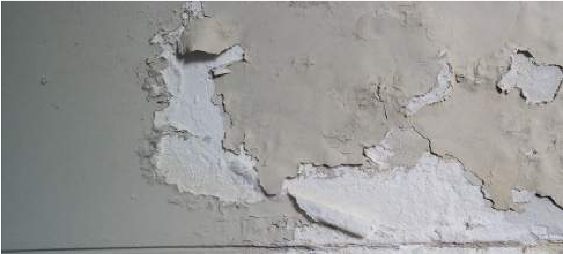
Figure 9.1: Ambulatory Wall. Joseph Newman, Fallin Steffen.
