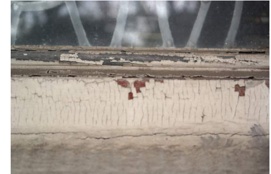
Figure 9.9: Blistering on Chapel Wall; Figure 9.10: Alligatoring on Exterior Window Frame. Joseph Newman and Fallin Steffen
