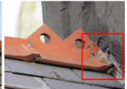
Figure 5.34-5.36 : Ridge tiles on the chapel; mortars and connections noted. Photo by Laura Stokley, 2015
