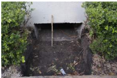
Figures 7.14 & 7.15: Exposed vents covered by a foot of soil during grade changes over time, photo by Amanda Keith, 2015
