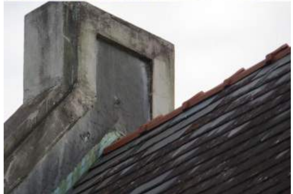
Figure 5.39-5.41 : Ridge tiles on the Freret and Wolf addition, also found on some parts of the Cathedral. Photos by Laura Stokley, 2015
