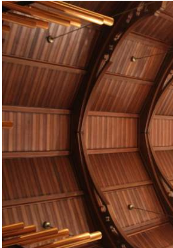
Figure 4.5: Cathedral ceiling. Photo by Cody Ellis, 2015.
