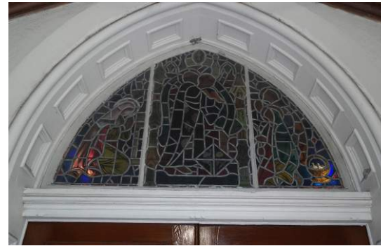
Figure 3.17: Non-vented window/transom at Cathedral main entrance.
