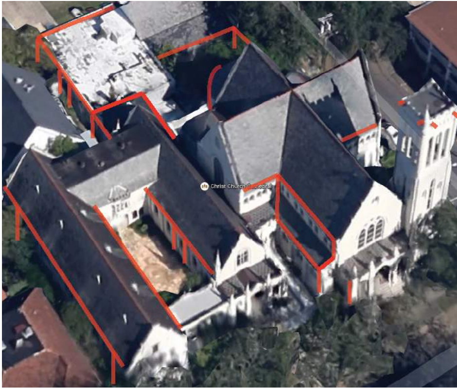
Figure # 6.4: On this aerial view of the church, gutters and downspouts are mapped in red. Photo by Google Earth, Edits by Nathan Lott, 2015
