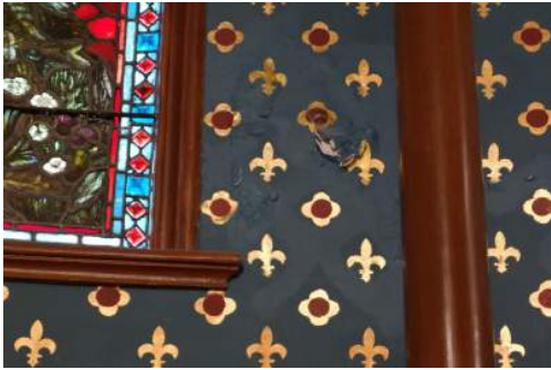
Figure 9.7: Blistering on Chancel Wall; Figure 9.8: Blistering on Vestry Wall. Joseph Newman and Fallin Steffen
