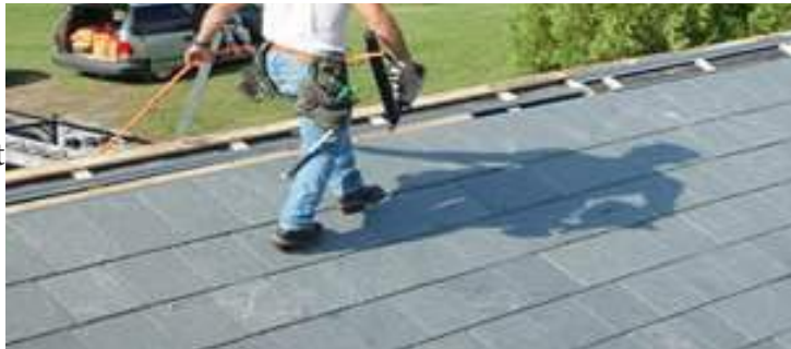
Figure 4.28: How to step on a slate roof Source: "How the Nu-lok Roofing System Works" Accessed March 4, 2015.
