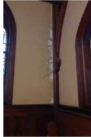
Figure 9.9: Blistering on Chapel Wall; Figure 9.10: Alligatoring on Exterior Window Frame. Joseph Newman and Fallin Steffen
