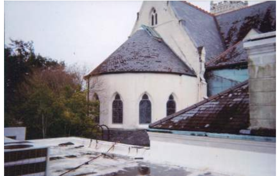
Figure 4.10: Apse roof. Courtesy of Dimitri Roby, 2014.
