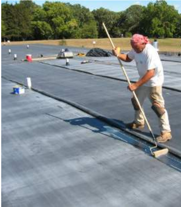
Figure 4.41: Application of sealant at seams of an EPDM roof Source: http://www.epdmroofs.org/what-is-epdm
