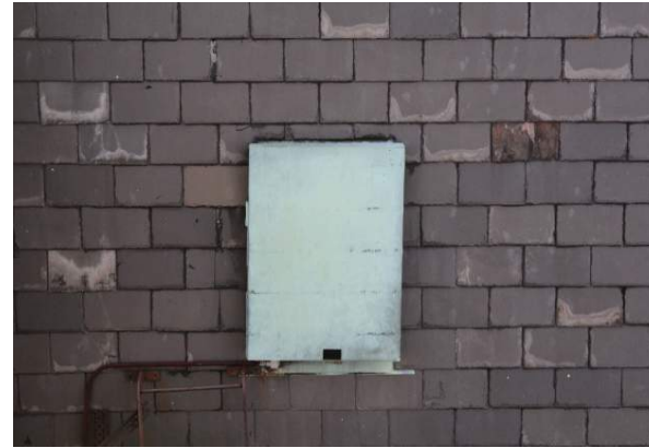
Figure 4.6: Entry hatch of the cathedral roof. Photo by Cody Ellis, 2015.
