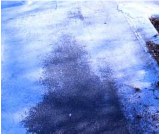
Figure 4.35: Current wear of reflective paint on roof Photo courtesy of Christine Carlo, 2015
