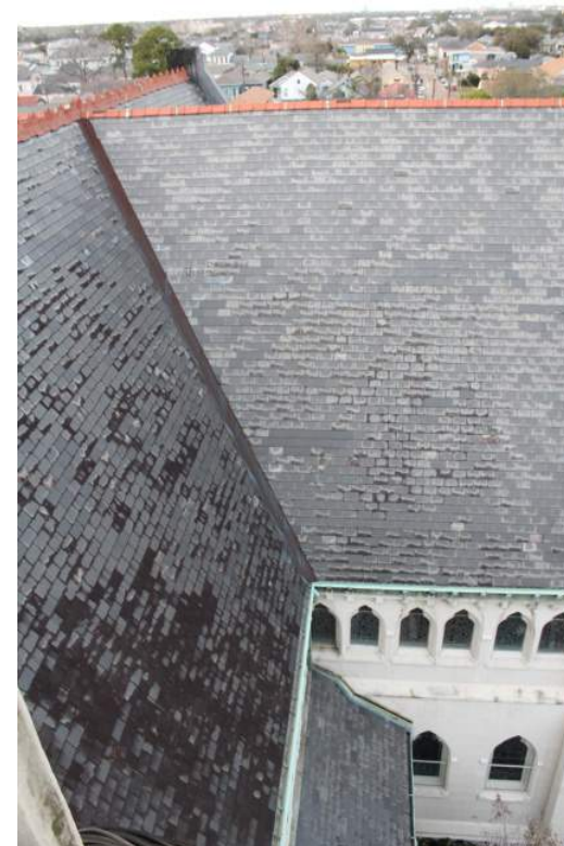
Figure 4.3: Ridge condition of the cathedral roof. Photo by Cody Ellis, 2015.
