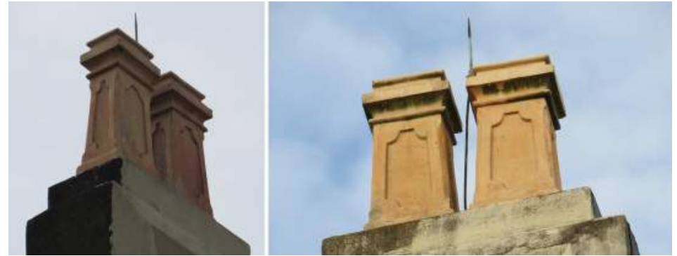
Figure 5.37-5.38 : Clay chimney tops on the cathedral. Photos by Laura Stokley, 2015
