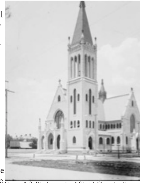
Figure 1.2: Photograph of Christ Church after completion. Courtesy of Louisiana State Museum
