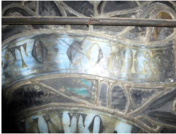
Figure 3.14: Cracks in window
