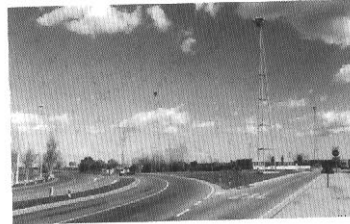
LEFT: View of existing site
