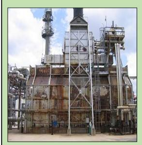
Furnace Improvements (FIS) was employed to carry out a capacity improvement of the Reactor Charge Heater (080-H-001). The client wanted to increase the process heat duty from 29.95 MMBtu/hr. to 37 MMBtu/hr. The maximum firing rate limitation was 54 MMBtu/hr.
