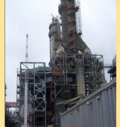
A refinery has a Crude Heater (191-H-1) in its Atmospheric Vacuum Unit AVU-191. The heater was built in 1969 and designed for 160,000 BPD at a total heat duty of 490.7 MMBtu/hr. The heater was later revamped to process 178,500 BPD of crude and 31,500 BPD of slip stream at total heat duty of 612.4 MMBtu/hr.
