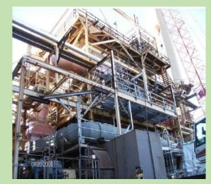
Furnace Improvements (FIS) was approached to convert a CO boiler in Unit 40 to be a standalone refinery fuel gas fired boiler, and reduce NOx emissions. The existing boiler was revamped into a fuel gas fired boiler with a maximum capacity of 400,000 lb/hr of steam @ 625 psig, 750 °F and reduced the NOx emissions down to 0.02 lb/MMBTU (16 ppm).
