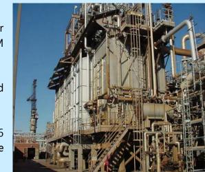
FIS carried out the entire scope of activities from conceptualization to commissioning of this heater revamp. The heater was successfully commissioned in October 2004. The NOx emissions were reduced to less than 0.03 lbs Btu.
