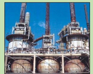
Furnace Improvements (FIS) was employed to re-rate Heater process using Low NOx Burners and increase the capacity on Platformer Heaters (H-4/5). The heaters were originally built in 1959. The heaters were changed to forced draft in 1977. Common air pre-heater, induced draft and forced draft fan were added to pre-heat the combustion air. Process fluid is heated in radiant sections. Convection section is used for steam generation.
