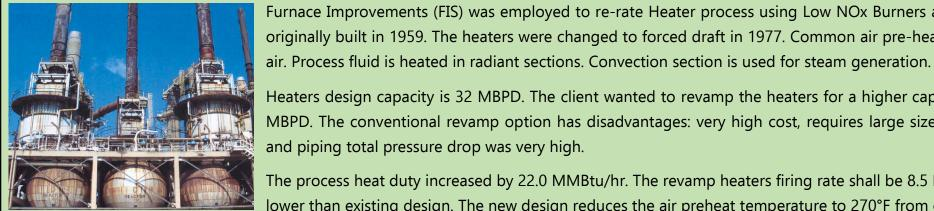
Furnace Improvements (FIS) was employed to re-rate Heater process using Low NOx Burners and increase the Capacity on Platformer Heaters (H-4 / H-5). The heaters were originally built in 1959. The heaters were changed to forced draft in 1977. Common air pre-heater, induced draft and forced draft fan were added to pre-heat the combustion
