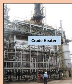
The client was already planning to install a new in-kind convection section, new stack, and a new tight shut-off damper during the forthcoming shutdown. FIS analyzed the design of the Crude Heater (11-F-01) and developed a scheme to increase the capacity and improve the efficiency of both Heaters.
