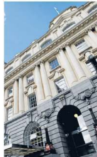
Second life: Britomart, in downtown Auckland, is now much more than a transport centre. Photo: ATEED
