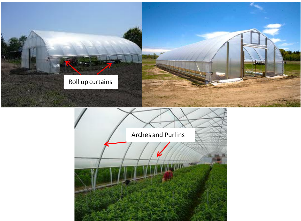
Polyethylene –Gothic arch
