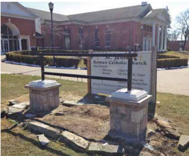
A steel structure stands during a dry before it's buried inside the panel and HDU posts to ensure the stone pillars were correctly positioned, level and plumb. Behind the new foundation is the sign it replaced.
