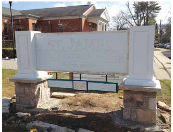
A dry fit is done prior to applying gold leaf to the lettering. This is done to confirm that the panel and posts all fit together as designed.
