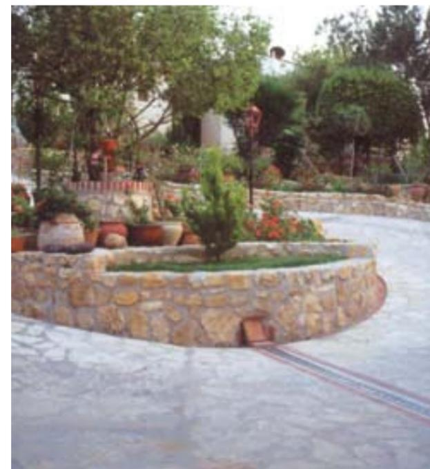
Figure 25: Paved areas directed to catch rainwater via a small collection channel.
