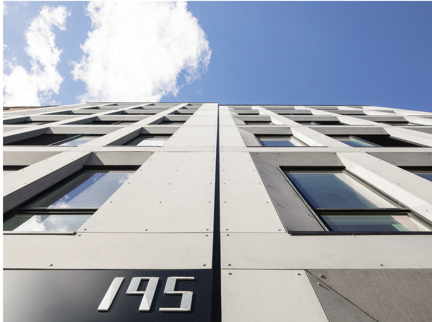
1 Street facade close up
