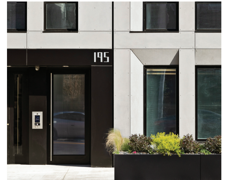
1 Street facade close up 1 Entry close up
