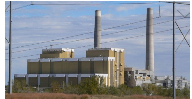
Gerald Gentleman Station (NE)
