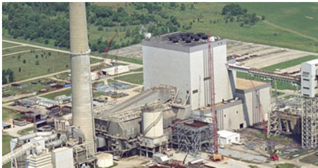
East Bend Generating Station (KY)
