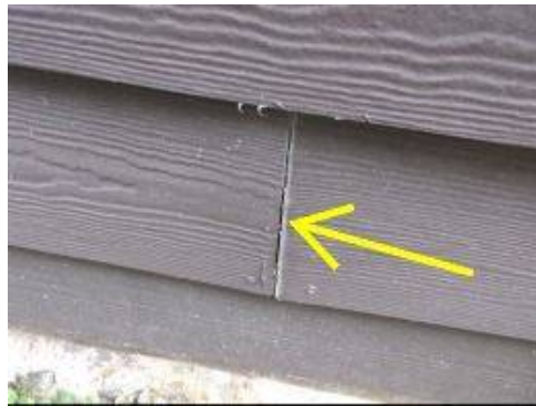
Photo 5-10 Caulk and seal all exterior butt siding joints.
