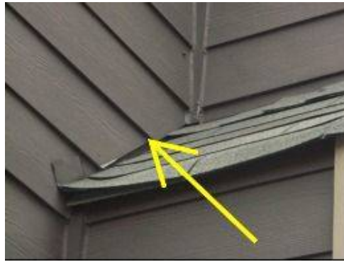
Photo 10-6 Flashing visible from rear yard.
