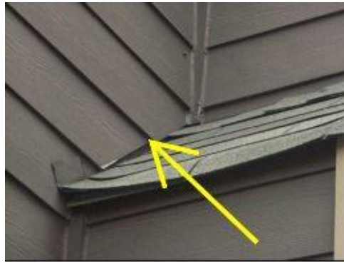
Photo 10-6 Flashing visible from rear yard.
