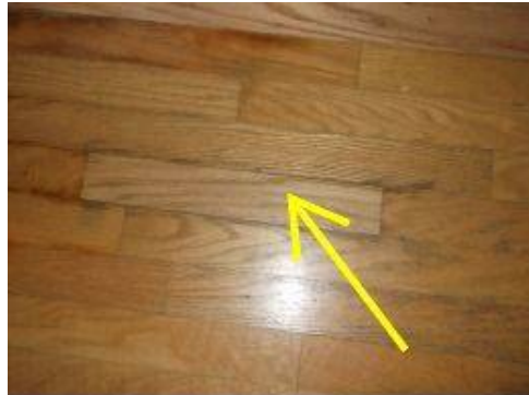
Photo 30-2 Laminate flooring in family room appears to have been repaired or a section replaced. Inquire of current owner or tenant if this is the case.
