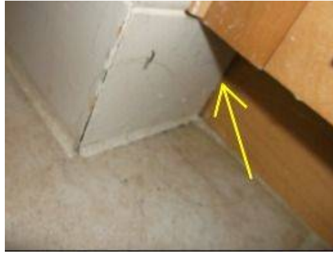
Photo 29-8 Seal spaces at the corners underneath bathroom cabinets.
