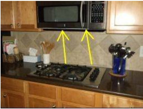
Photo 28-5 The distance between the burner elements on the surface unit is approx. 18 inches from the bottom of the microwave and exhaust filters. Exercise due caution when using the surface unit burners. Kitchen fires often start from this area.
