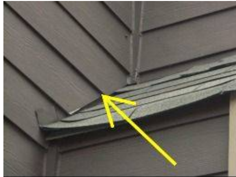
Photo 10-6 Flashing visible from rear yard.
