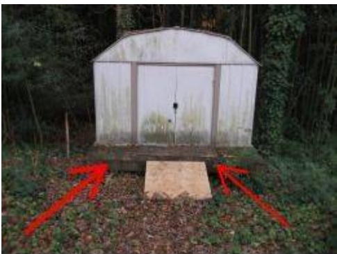
Photo X-9 Outbuildings are excluded from this inspection, however, it should be monitored such that small children do not become entrapped. Also the space underneath is an excellent harbor for rats and snakes. You want to consider installing skirting around the wooden support foundation.
