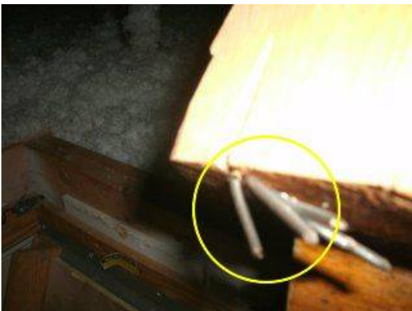
Photo X-7 POTENTIAL SAFETY HAZARD. NAILS ARE PROTRUDING AT ENTRANCE TO ATTIC STAIRS....INVITING INJURIES. EXERCISE CAUTION WHEN ENTERING AT THIS LOCATION. REPAIR AS SOON AS PRACTICABLE.
