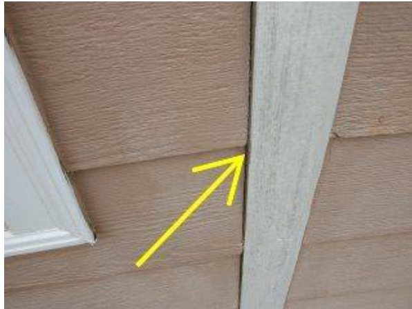
Photo X-6 SEAL ALL EXTERIOR SIDING JOINTS.
