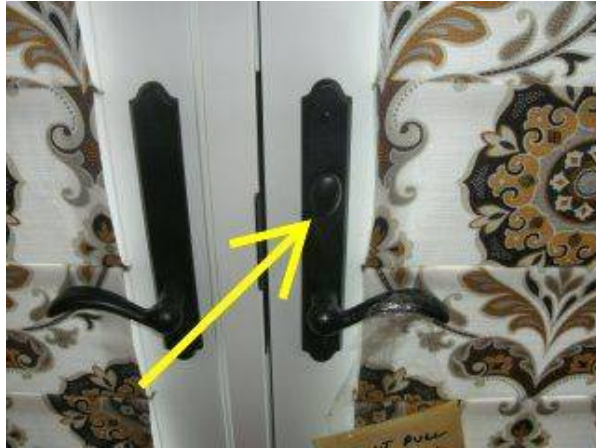
Photo X-12 DOORS SHOULD NOT REQUIRE THE USE OF A TOOL, SPECIAL KNOWLEDGE OR KEY TO GAIN EXIT IN AN EMERGENCY.
