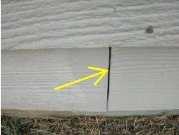
Photo X-11 GAPS IN EXTERIOR SIDING NEED CAULK AND SEALED WITH WEATHER-RESISTANT TYPE CAULK.
