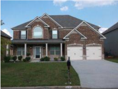
Photo X-1 Front entrance view from Dinmont Chase.
