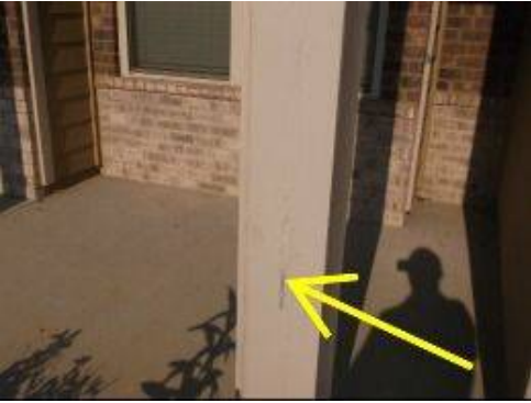
Photo X-11 Front porch support columns need re-painting with prime plus 2 coats of premium quality paint. Wood members are exposed to the weather. Re-paint where necessary.
