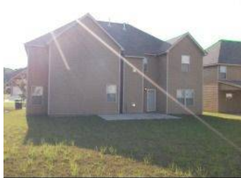
Photo X-42 Rear view of 4070 Dinmont Chase.
