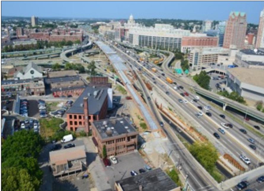
This project will replace the heavily-used I-95 Providence Viaduct in downtown Providence, including two 4-lane bridges that pass over the Woonasquatucket River, Amtrak's Northeast Corridor, and other ramps and local roads. Built in 1964, the bridge has surpassed its design life and is showing signs of aggressive deterioration.
