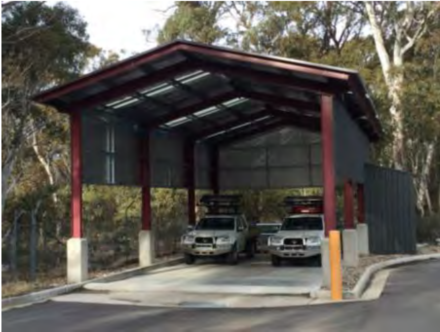
Bunded wash down bay
