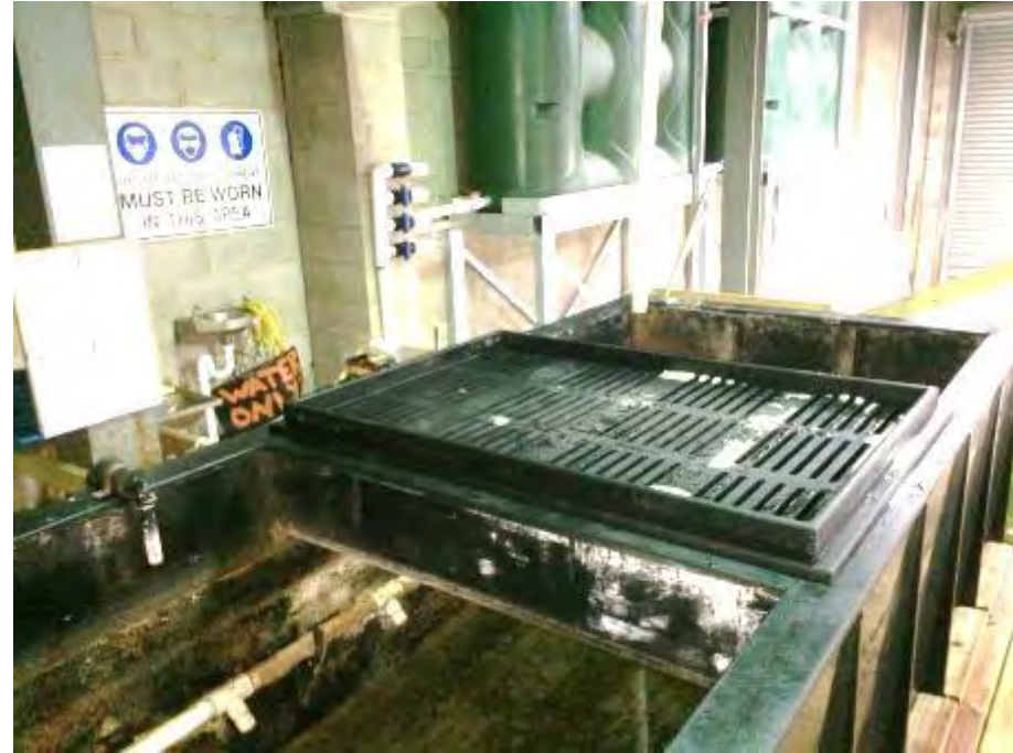
Wet Salt Batching tank
