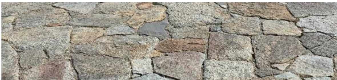
Figure 2: Example of stone-paved surface similar to intended upgraded Summit Walk track surface
