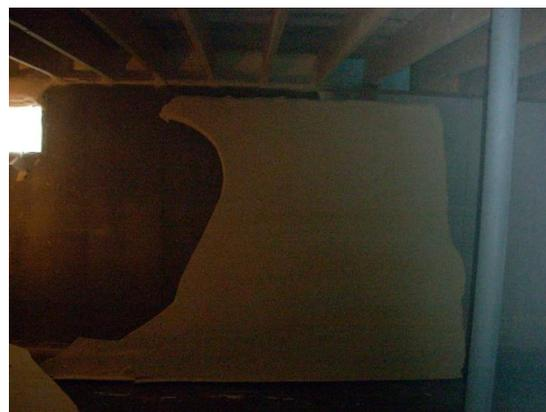
*Foam peeling off a foundation wall, in this case it came off as one big sheet.*
