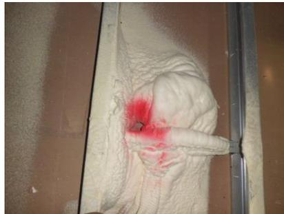
*The location marked in red paint shows where foam was sprayed over an electrical box but did not grow together to completely seal over the box.*
