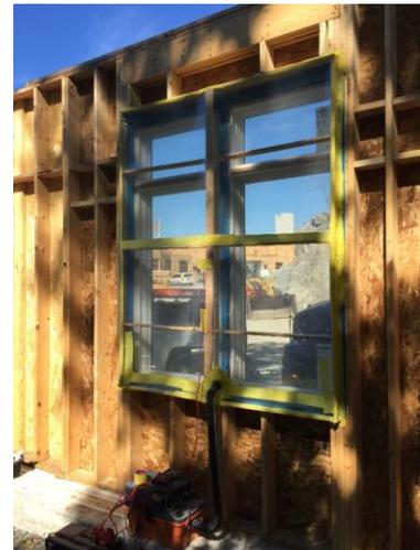
The test can be performed during multiple stages of the mock-up's construction for comparison, such as at "air barrier stage" and at "finish stage." If issues arise, the product can be retested until a solution is discovered and the solution can then be applied to the actual installations on the building itself. The images provided in supplement to this article illustrate a typical ASTM E1105/AAMA 502 test being performed on a stand-alone mock-up unit on a recent project of ours.
