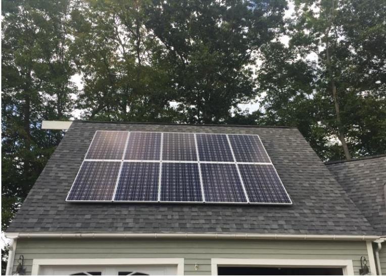
*Our PV array is just under 3.5kW and is comprised of ten (10) 72-cell modules. It's sized to produce 120% of our annual needs.*
