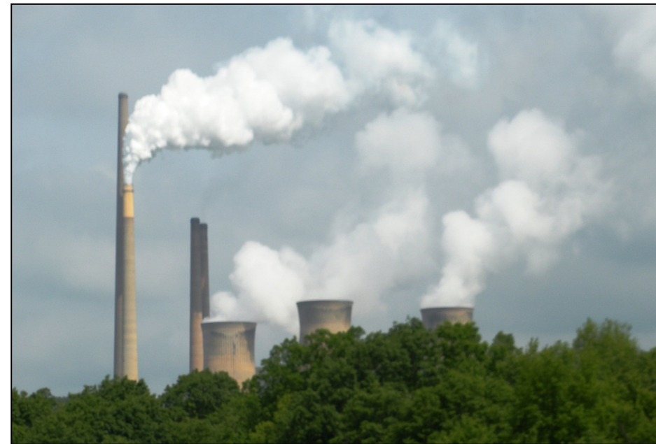
Photo 1: The Keystone Generating Station, Shelocta, PA, Armstrong County.
