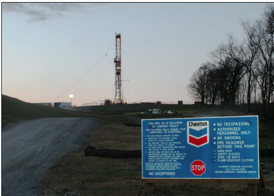
Photo 2: Shale Drilling Pad Site, Crabtree, PA, Westmoreland County.
