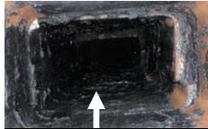
Creosote is a dark, sticky substance that is highly flammable shown inside of this chimney.
