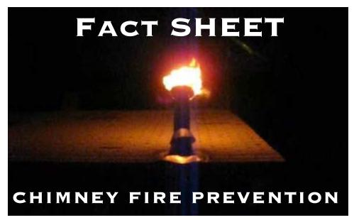
According to the latest statistics available, there are over 25,000 chimney fires per year in the US that are responsible for approximately 125 million dollars in property damage. Built up creosote is responsible for many of those fires, along with deficiencies in chimney linings and structures that allow high temperatures, embers and sparks to reach combustible areas that are adjacent to your chimney or fireplace.
