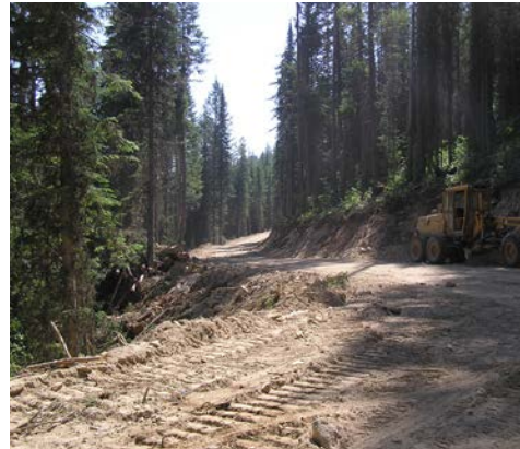
Properly constructed road in Inchelium District.
