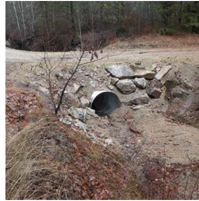
New 84" culvert on Owhi Creek
