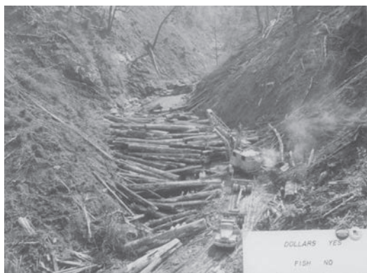
Historic, damaging logging road built in a stream.
