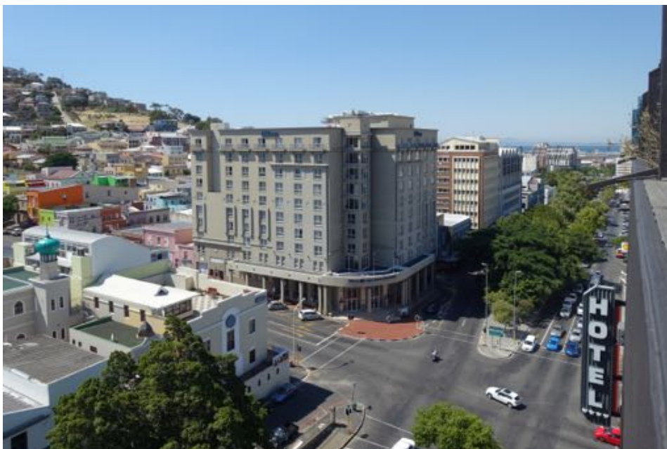
Figure 9: The view looking north up the Buitengracht: a further view that underscores the ham-fisted, insensitive, engineering-dominated insertion of the ‘thorn-like’ multi-storey wall of development between Rose Street and the Buitengracht, in contrast to the single and two-storey type of development that characterises the Bo-Kaap. For many residents of the Bo-Kaap this has meant that they have lost the views of Table Mountain and Devil’s Peak (author’s photo, January 2016).
