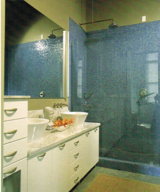
The walls and floors of the bathroom showers for Phase I of the Avenue Lofts project are ornamented in Hakatai Ashland Series MG001 1- x 1-inch Crystal Blue gloss tiles.
