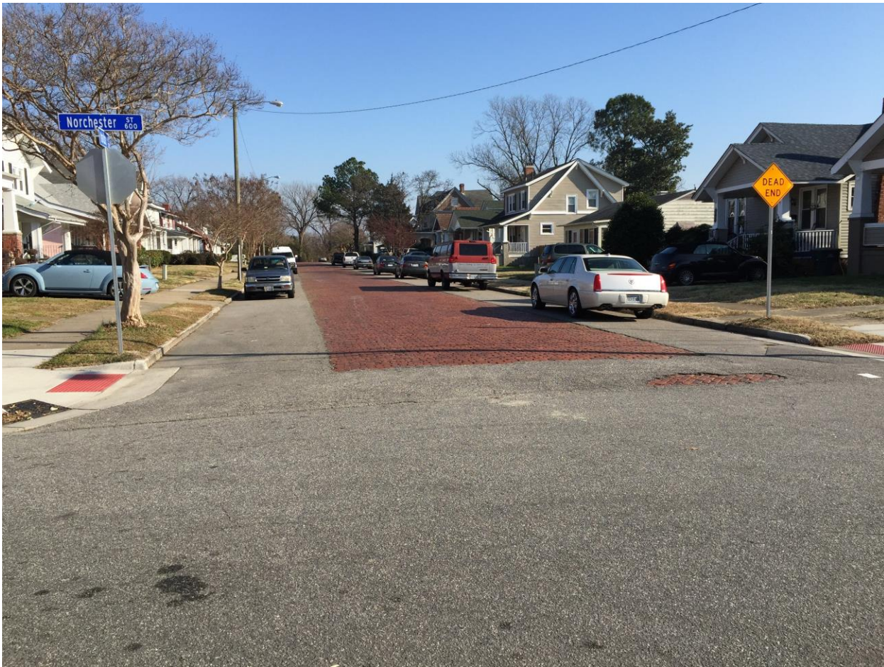
Marlboro Avenue Brick Pavers, Chesterfield Heights
