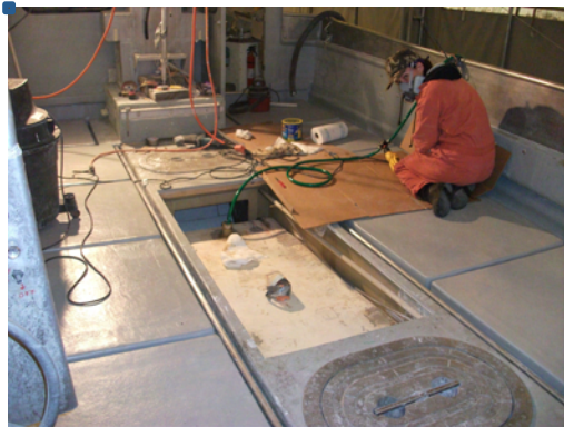
Figure 3: Just prior to 200-gallon tank removal
