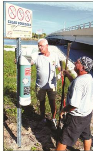
Peter Tomaszewski and Joe Spirito, both with Sanibel's Department of Public Works, installing a new Clear Your Gear station at Blind Pass
